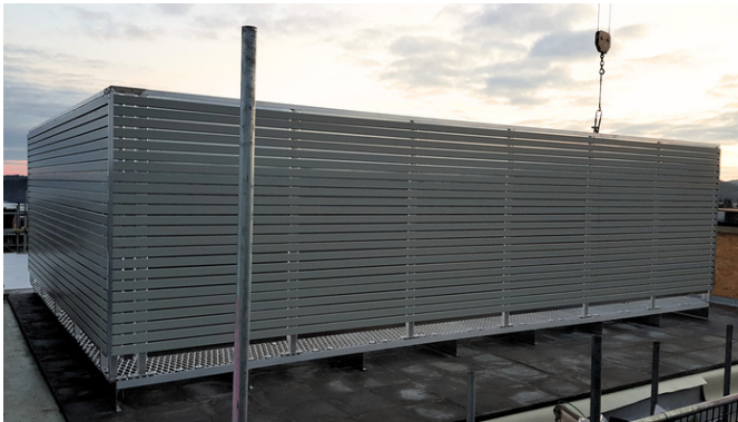
Acoustic Soundshield Screen to 2 sides with Greening Grey R510A05 powder coated slats
