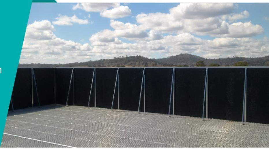
Acoustic+ combines the sound attenuation properties of both Soundshield and Peacemaker to yield superior noise reduction results. Actively reducing noise in three phases (absorbing – reflecting – absorbing), Acoustic+ is Configured Platforms premier acoustic solution. With a Weighted Sound Reduction Index  $Rw33dB$  and a Noise Reduction Coefficient (NRC) of 1.0
